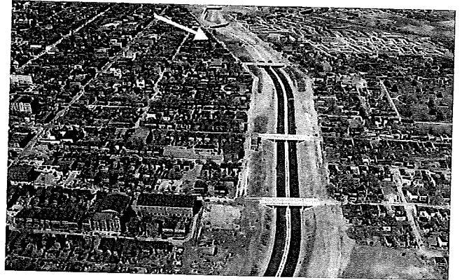
The Richmond-Petersburg Turnpike cut a trench one block wide and eighteen blocks long through Jackson Ward, destroying nearly 1000 homes in the historic center of Richmond's African American community. The highway avoided Sixth Mount Zion Church (top picture and arrow in bottom picture), the only surviving building on the north side of Duval Street. Top picture, taken November 3, 1957, is reprinted from the Richmond Times-Dispatch by permission.
